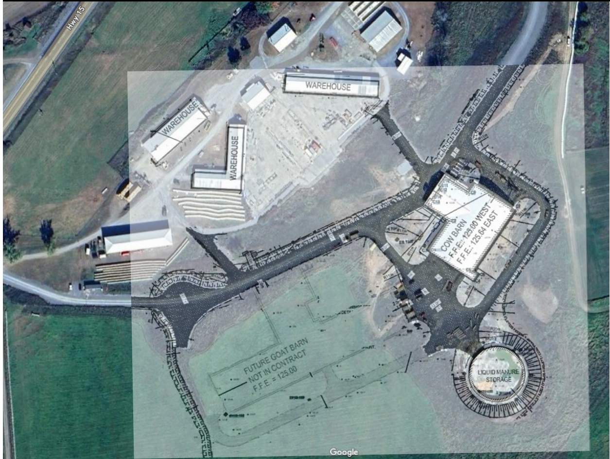
JOYCEVILLE FARM CONSTRUCTION SITE 2024 SUPERIMPOSED WITH ENGINEERING PLAN
