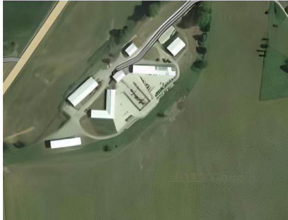
JOYCEVILLE FARM PRE-CONSTRUCTION 2022
