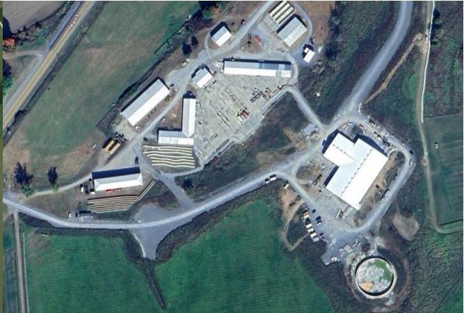
JOYCEVILLE FARM CONSTRUCTION SITE 2024
